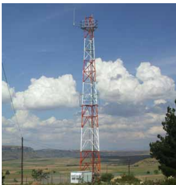
Rural communications infrastructure
