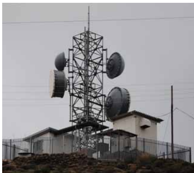
Rural communications network infrastructure
